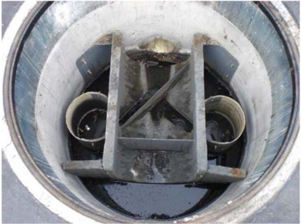
Inclined Outlet Screen Type 304 Stainless Steel 0.1875 in / 4.76 mm Staggered Round Performances
