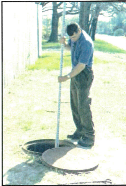
Sediment inspection using a stadia rod
